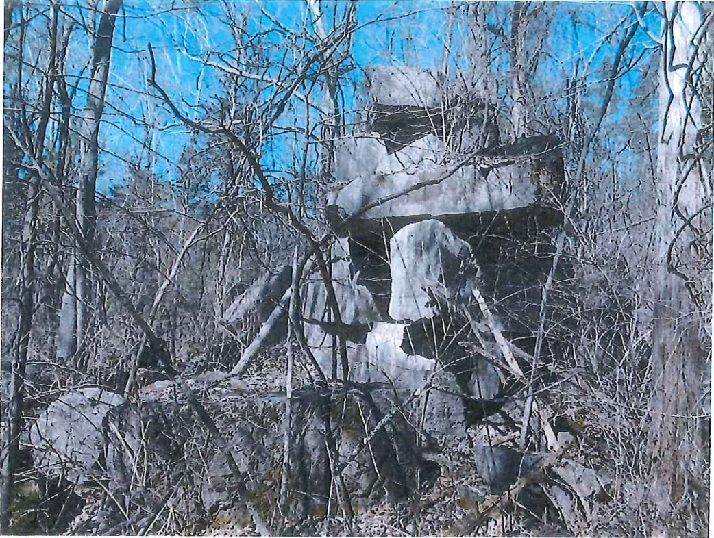
Fig. 4 This was the tallest pile of grout pile.
