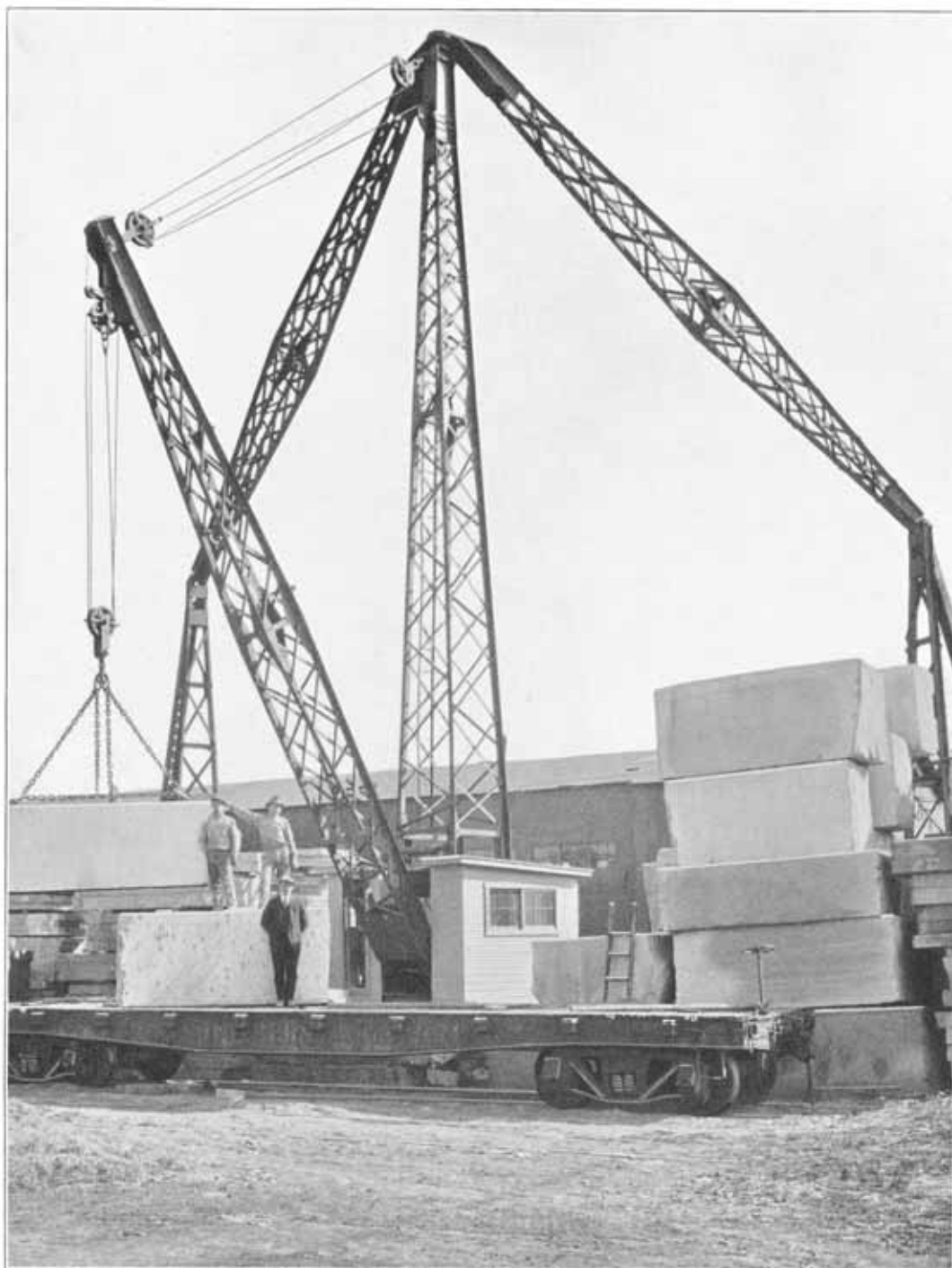
20-ton Self-Contained Complete Circle Stiff-Leg Derrick, Rowat Cut Stone Company, Des Moines, Iowa
