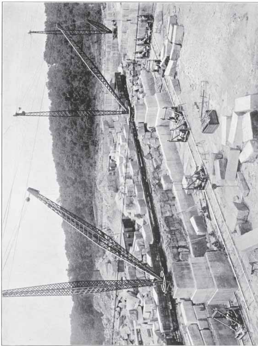
Eight Bedford Electric Wardwell Channeling Machines in Operation at Dark Hollow Quarry, Bedford. Also three All Steel 30-ton capacity Steel Derricks
