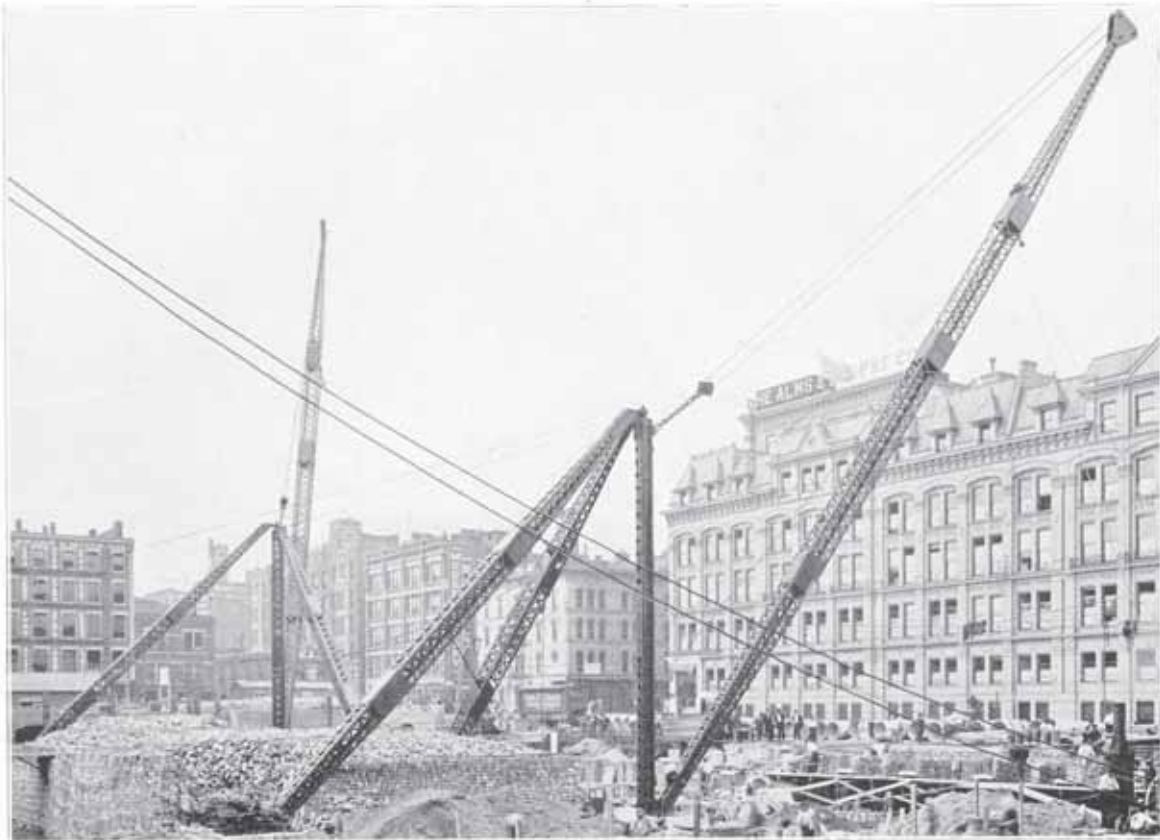
View of two Bedford Stiff-Leg Steel Derricks on construction work. These derricks are of 20-ton capacity, having 40-foot masts and 100-foot booms
