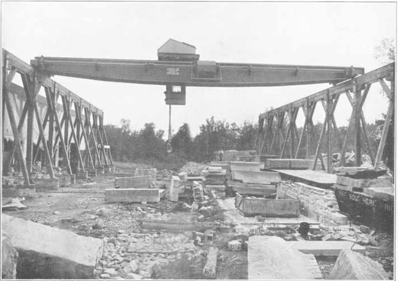
Shea & Donnelly Company, Bedford, Indiana, using a thirty-ton two-motor 70' 0" Span Bedford Electric Traveling Crane
