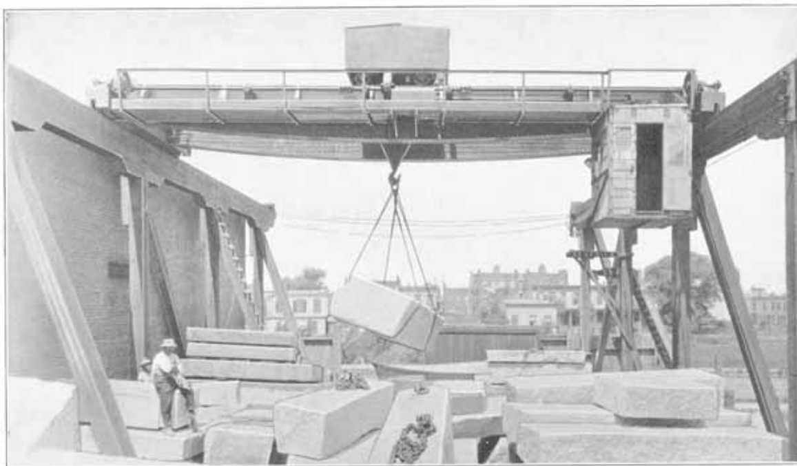
Tedeschi & Tedeschi, Long Island City, New York. 20-ton 39' span three-motor Electric Crane
